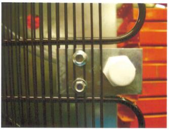
**14)** Fit the Drain Bracket to the condenser & secure with 2 screws.
