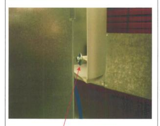
15) Replace the Side Panel by sliding slotted key hole over the screw shown (inside front panel) & guide the bottom slot into the moulded Base. Now secure using 3 screws as before.
