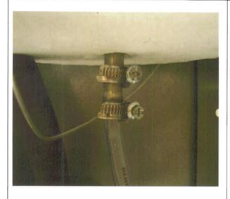
13) Push the Drain assy onto the Tank until it touches the insulation. Tighten the 2 Hose Clips having one <u>above</u> & one <u>below</u> the bump on the Stainless Steel pipe.
